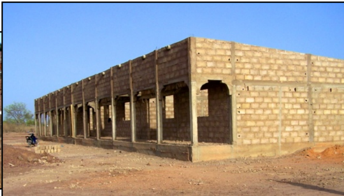
Four classroom building April 2014
