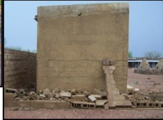
A large section of the enclosing wall fell down and the guard house next to it suffered several cracks in the walls. Temporary thatch wall was put up to keep animals out of the yard.
