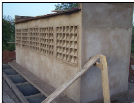
Rear view of latrines
